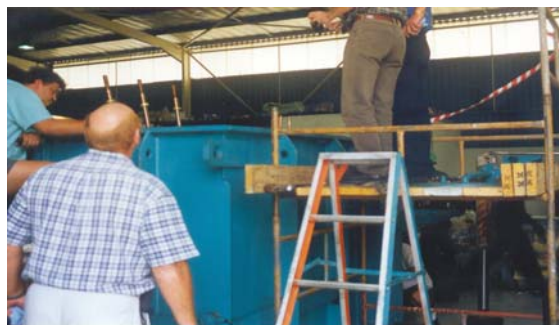
Figure 15-Reactor transformer being De-tanked at the Works facility
