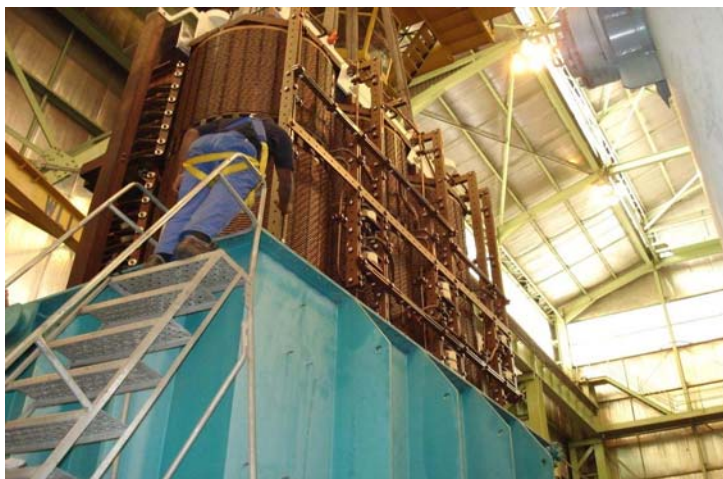
Figure 28-Transformer De-tanking
